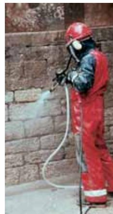
Wide range whirl blaster system OERTZEN TORNADO - for abrasive surface treatment, paint removal, de-rusting, and concrete restoration.
